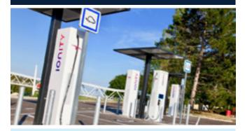
In late 2019, 16 very high power electric charging stations were added to the APRR and AREA network. Powered entirely by electricity from renewable energy, these can reduce the charging time of vehicles to about 10 minutes, compared to 30 minutes on the existing high power terminals, or nine hours via a home outlet.
