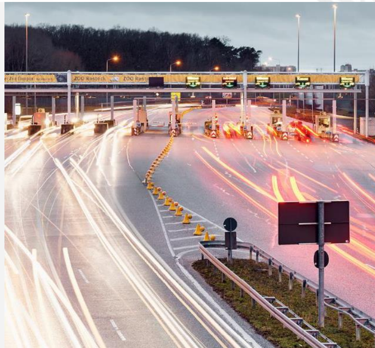
Photo of Warnow Tunnel, source: Trent Perrett Photography
